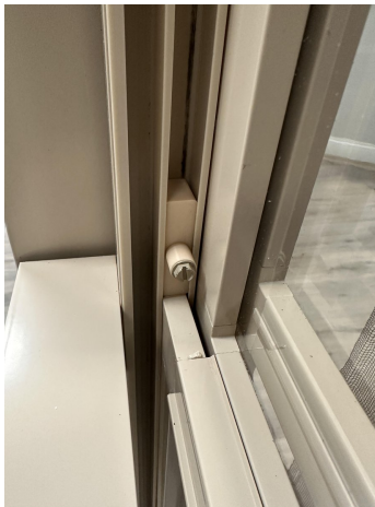
Fig. A.4.5: Vent Lock in sash track
