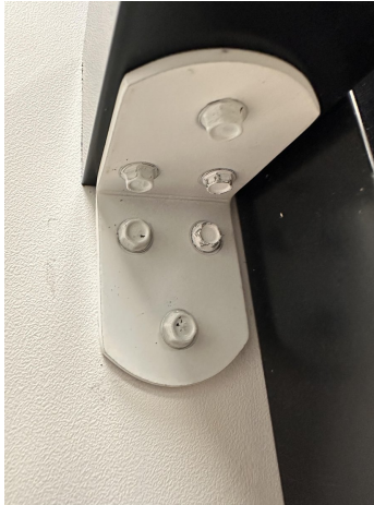
Fig. A.4.4: Fall rail mounting bracket
